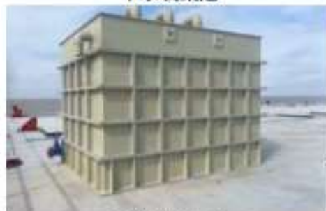
码头油污水罐
